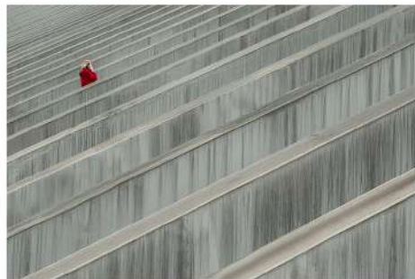
Open - Between concrete
